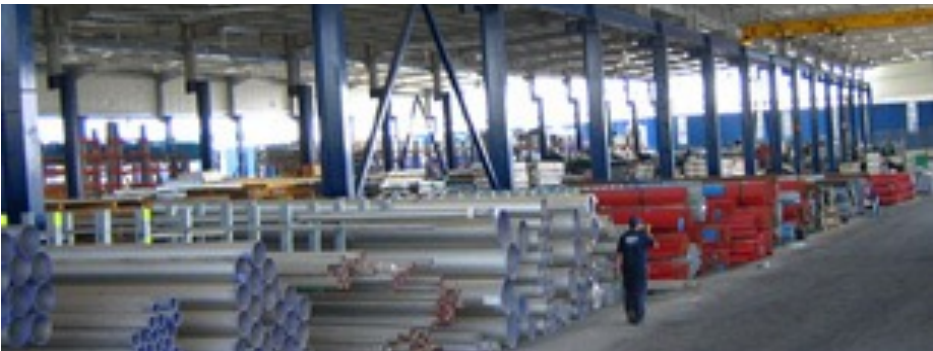
Figure 5 - Shed Storage Facilities
