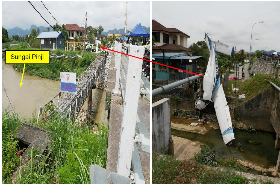
Figure 17: Final position of aircraft at the water diversion culvert beside Sungai Pinji.
