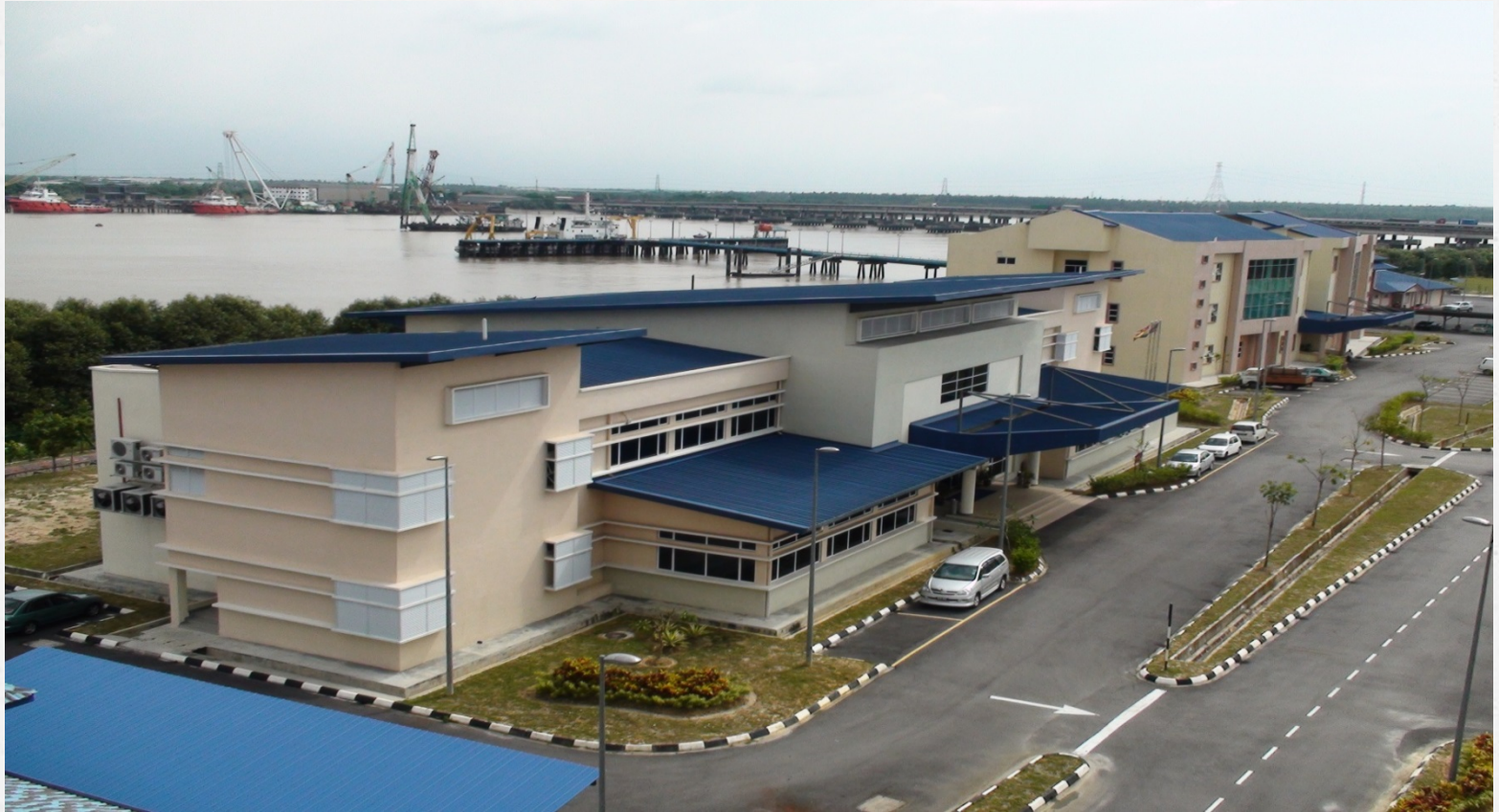
Training Centre Bulding
