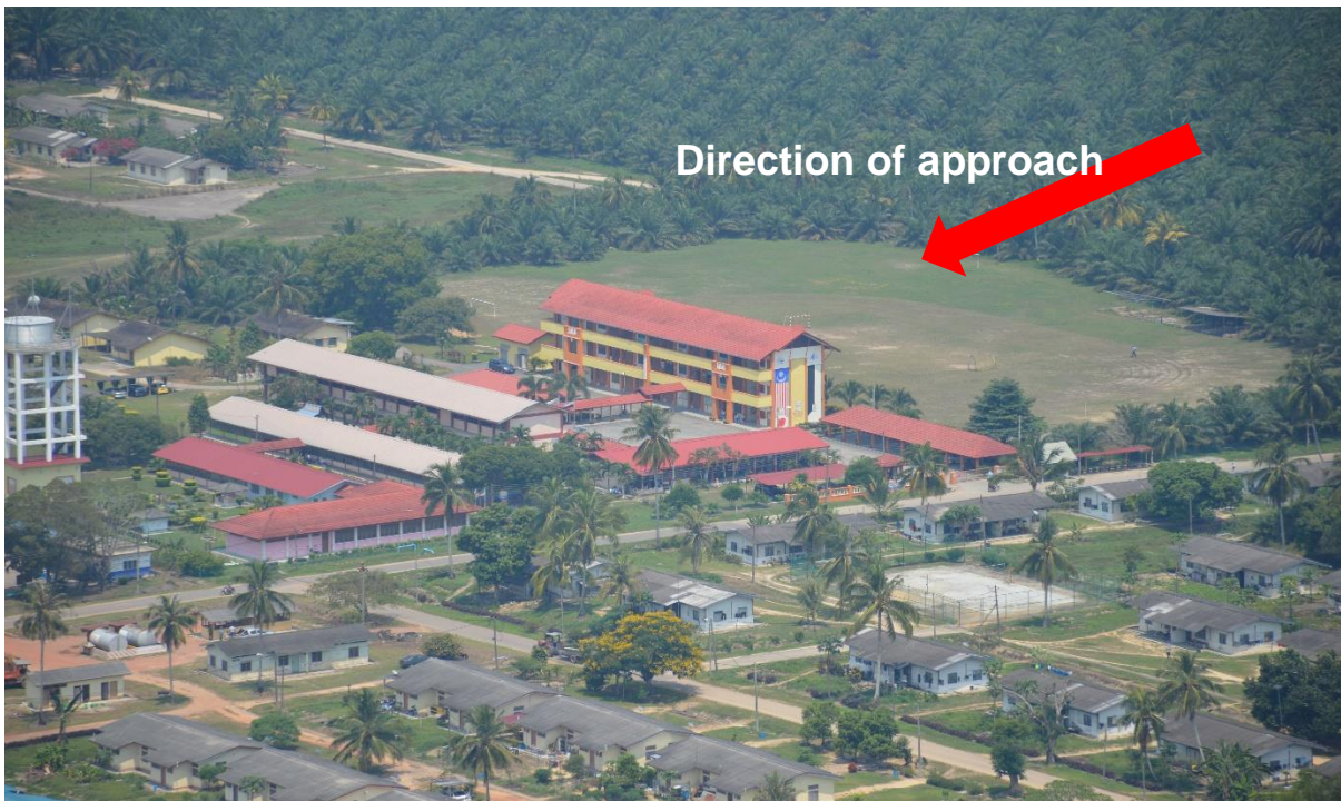
Direction of approach before landing
