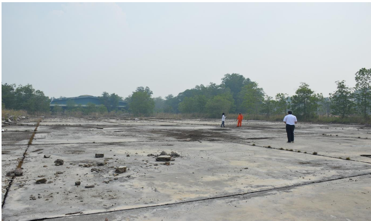
Cemented area of abandoned factory
