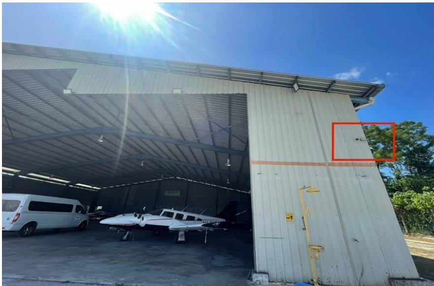
Figure 33: CCTV Camera location
