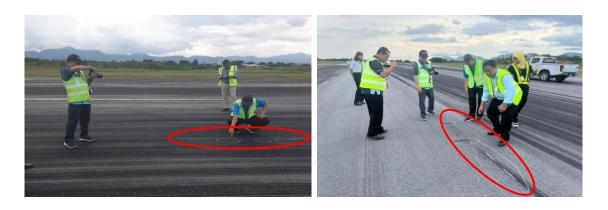
Figure 12: Scratched marking from the propeller on the runway during the hard landing.
