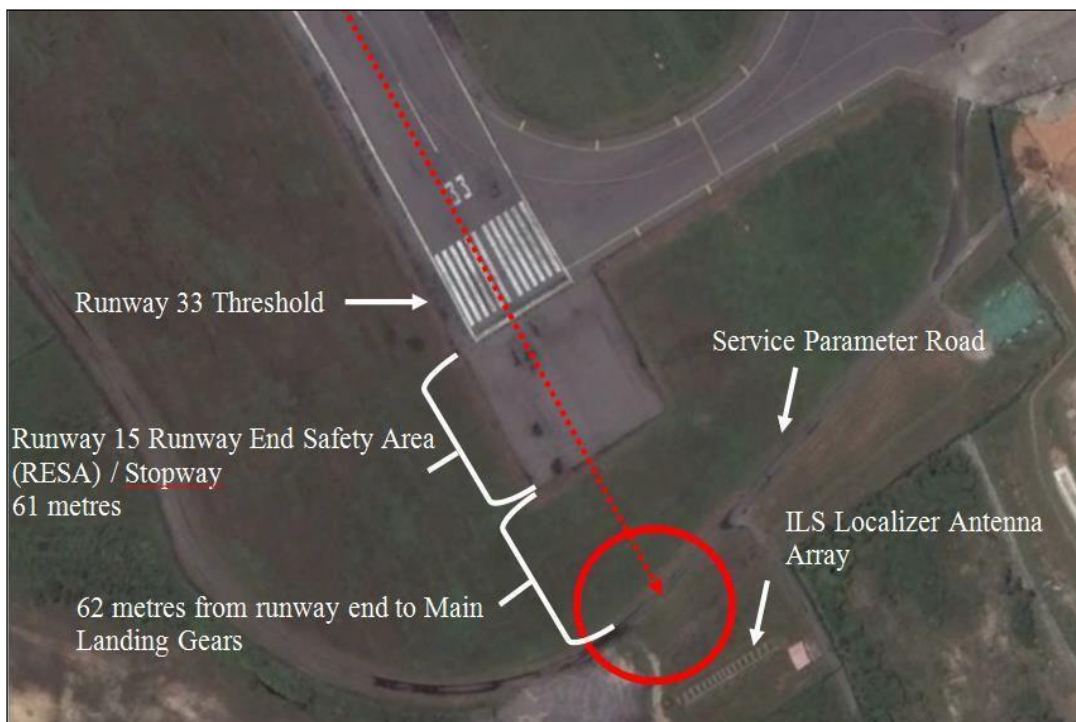
Figure 57: Zoom in of impact area at the end of runway 15
