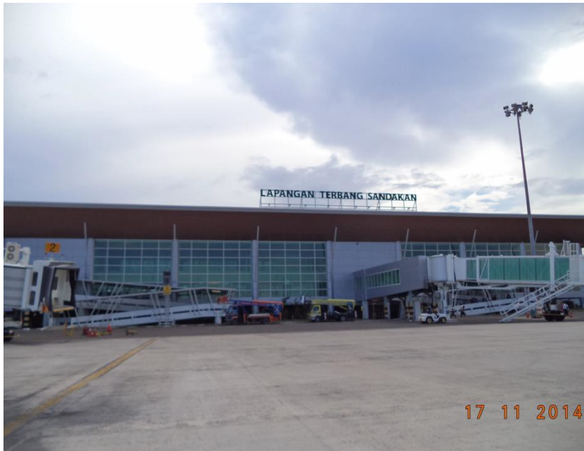
Picture after completion of upgrading works (airside view)
