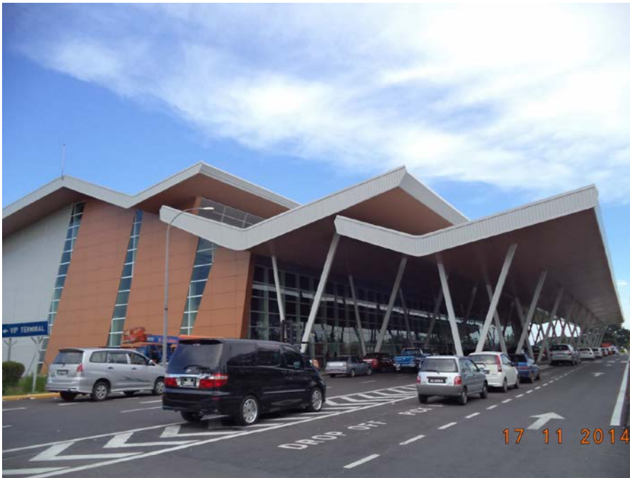
Picture after completion of upgrading works (landside view)
