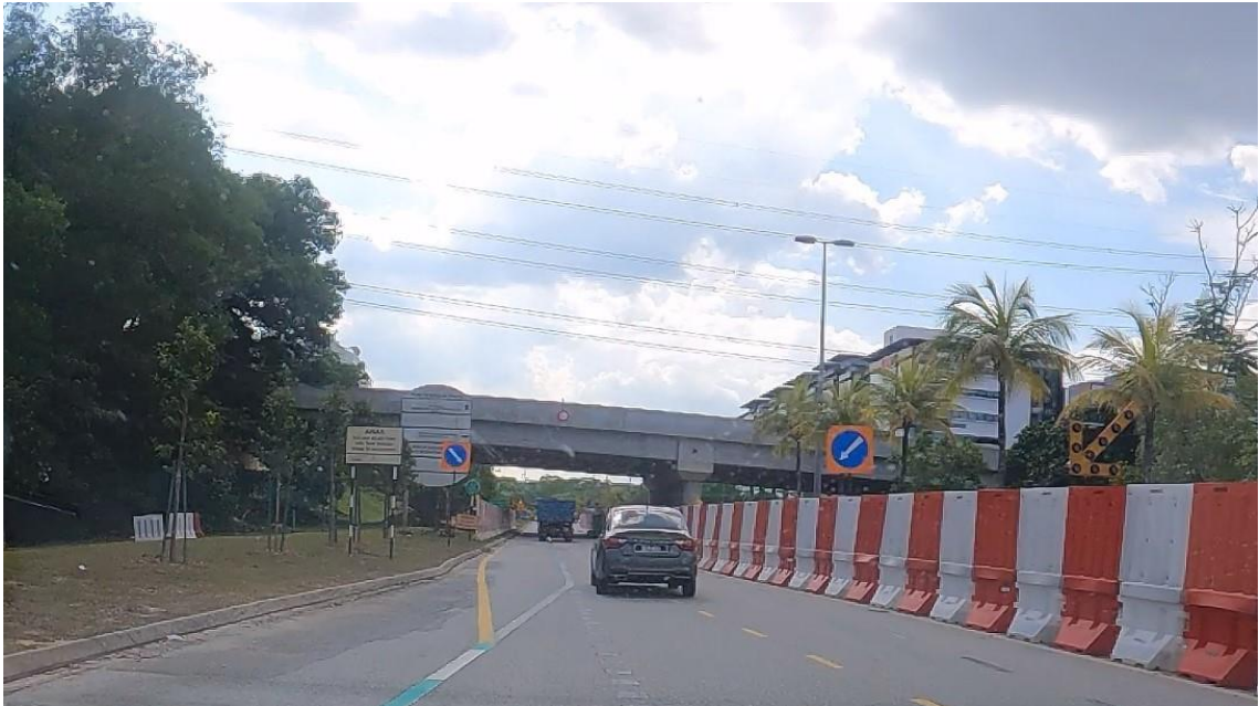
Figure A.6: Route B road conditions in Cyberjaya
