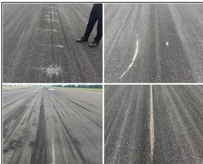
Figure 3: Scrape marks on the Runway
