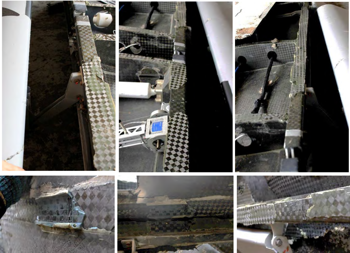
Figure 6. Skin/Spar Failure Mode
