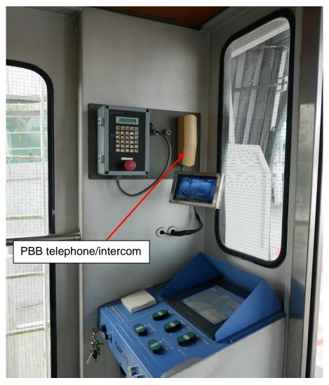
Figure 22: PBB Telephone/Intercom at PBB Operating Console
