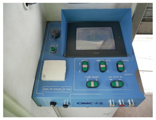
Figure 20: PBB Operating Console LCD Touch Screen Display PBB Bay 1
