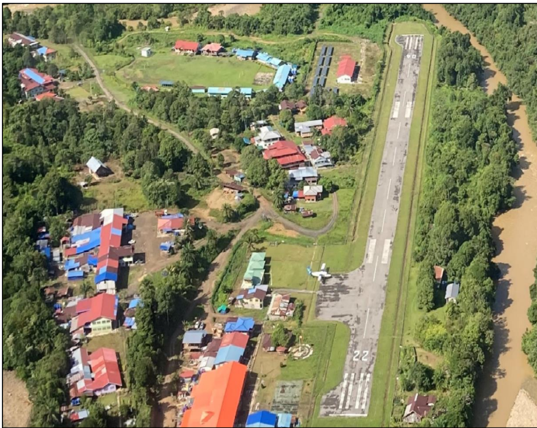
Figure 31: Site reconnaissance and mapping on Long Seridan runway using DJI Phantom 4 Pro Version 2.0 Drone
