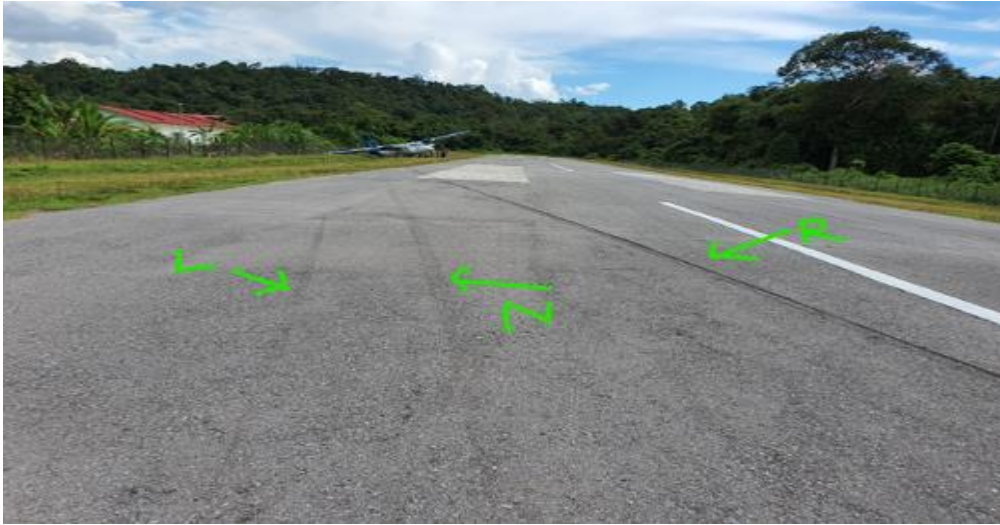
Figure 52: Photograph of the runway taken after the incident showing the tyre marks of the aircraft
