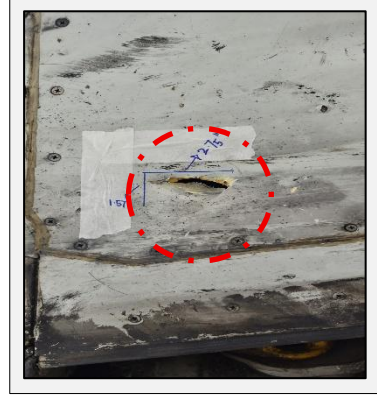
Figure 14: RH Lower Panel Main Landing Gear Ruptured
