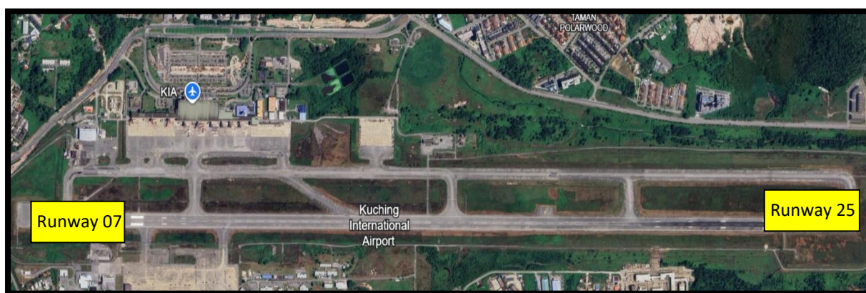
Figure 2: Aerial Overview of Kuching International Airport (WBGG)
