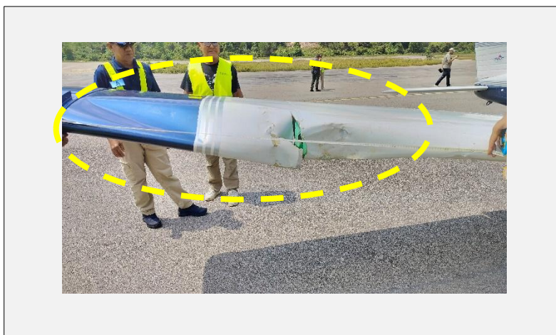
Figure 4: Front View – Structural condition of the RH Wing Leading Edge
