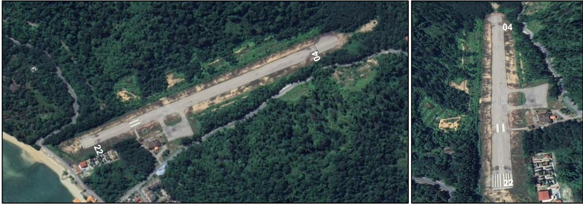
Figure 9: Aerial view of Pangkor Island Airport
