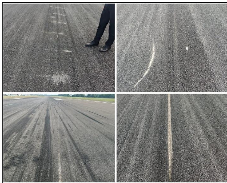
Figure 8: Scrape marks on the Runway
