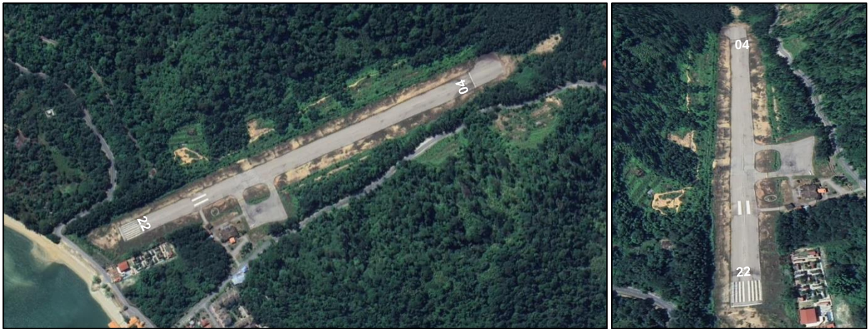
Figure 9: Aerial view of Pangkor Island Airport
