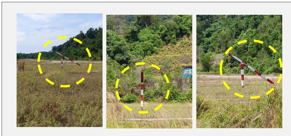
Figure 8: The windsock at the aerodrome was found broken and unserviceable condition.
