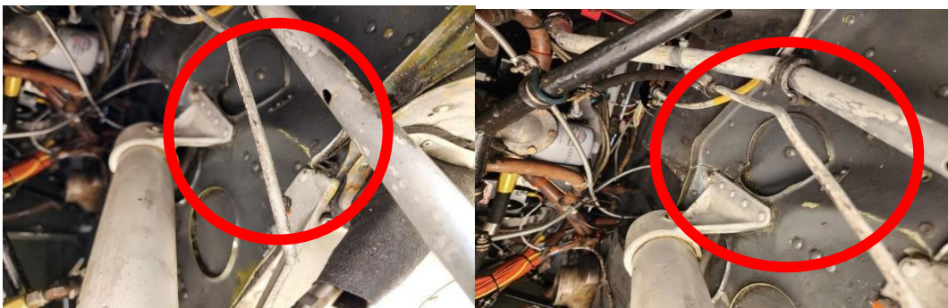
Figure 3: Buckled and damage
