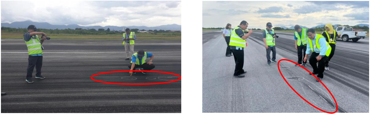
Figure 12: Scratched marking from the propeller on the runway during the hard landing.
