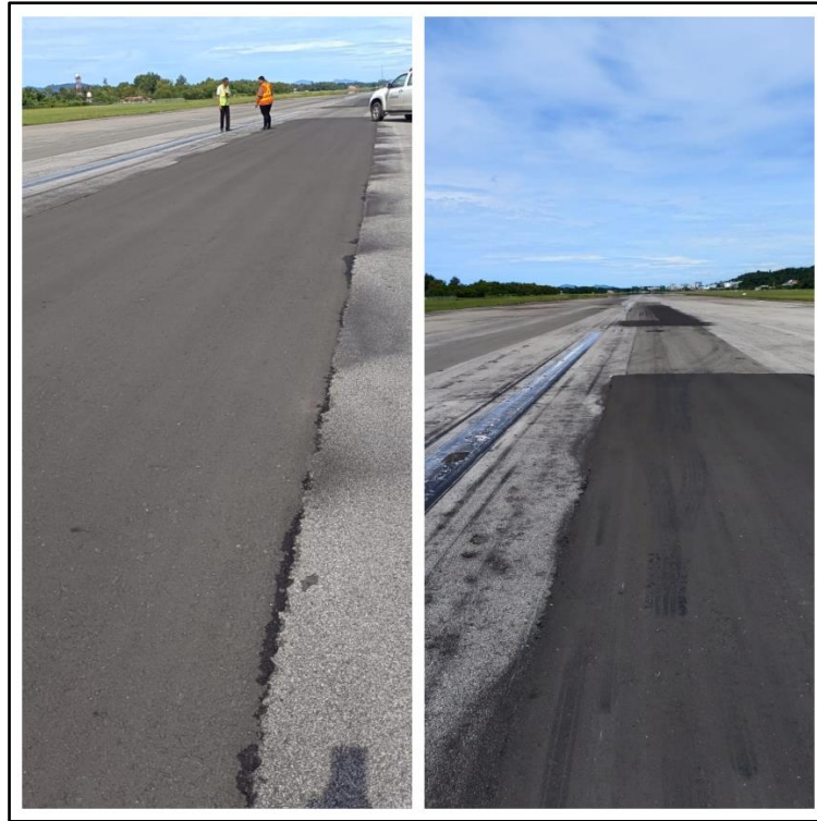
Figure 7: New big patch was applied but the joint at the side between the new and old started to dislodge gradually
