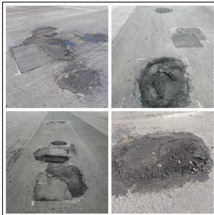
Figure 6: Peeled-off runway surface from temporary patchwork
