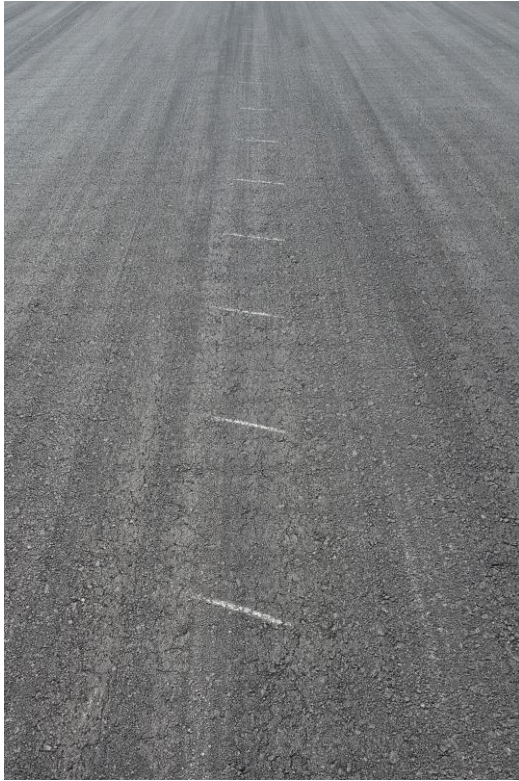
Photo of skid marks on runway
