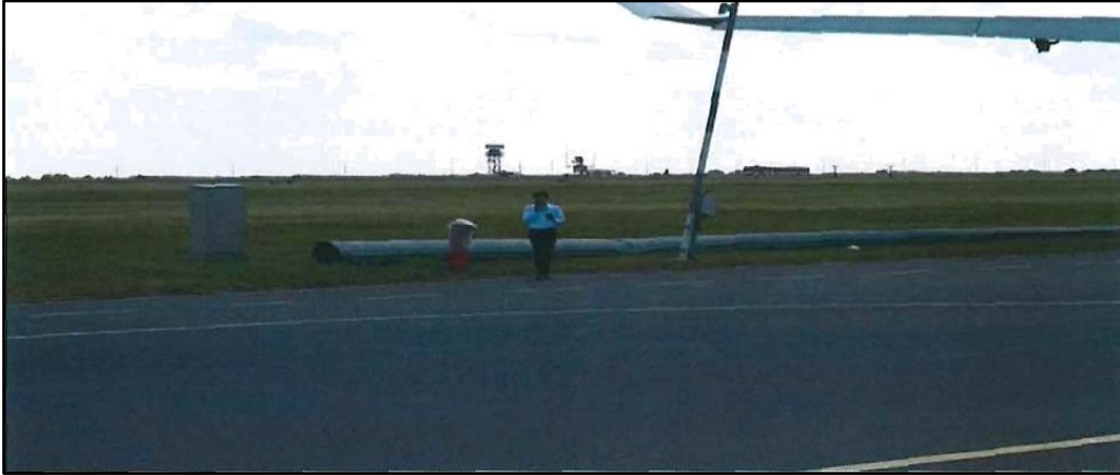
Figure 6: Light pole lying on floor and CCTV pole slanted
