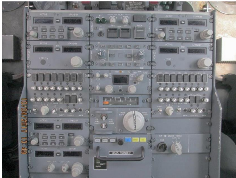
Figure 11: Photograph of Center pedestal
